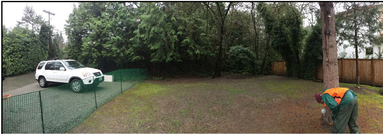
Photo 4: Compacted area with tree protection fencing in place. Tree #3 in foreground on right.
